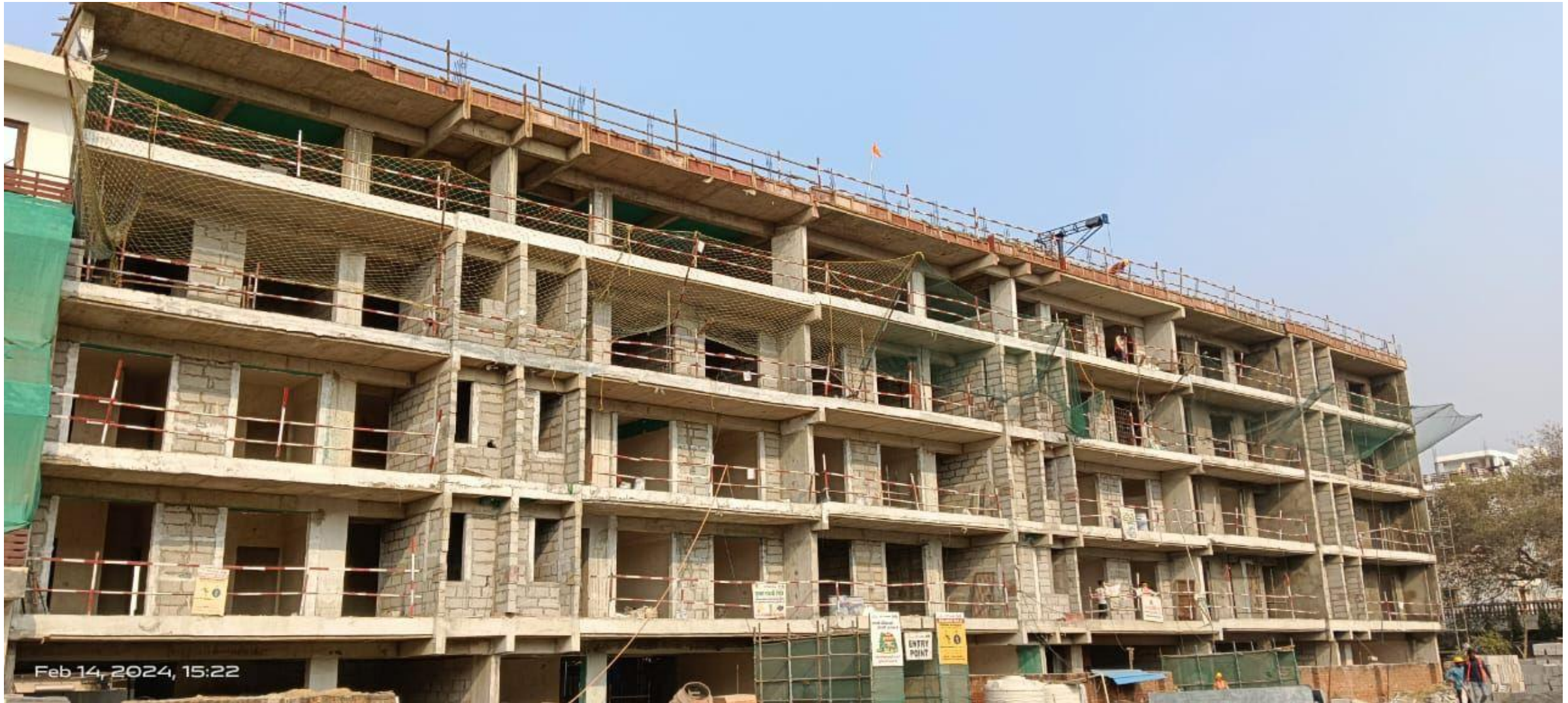
Sub & Super structure WIP
